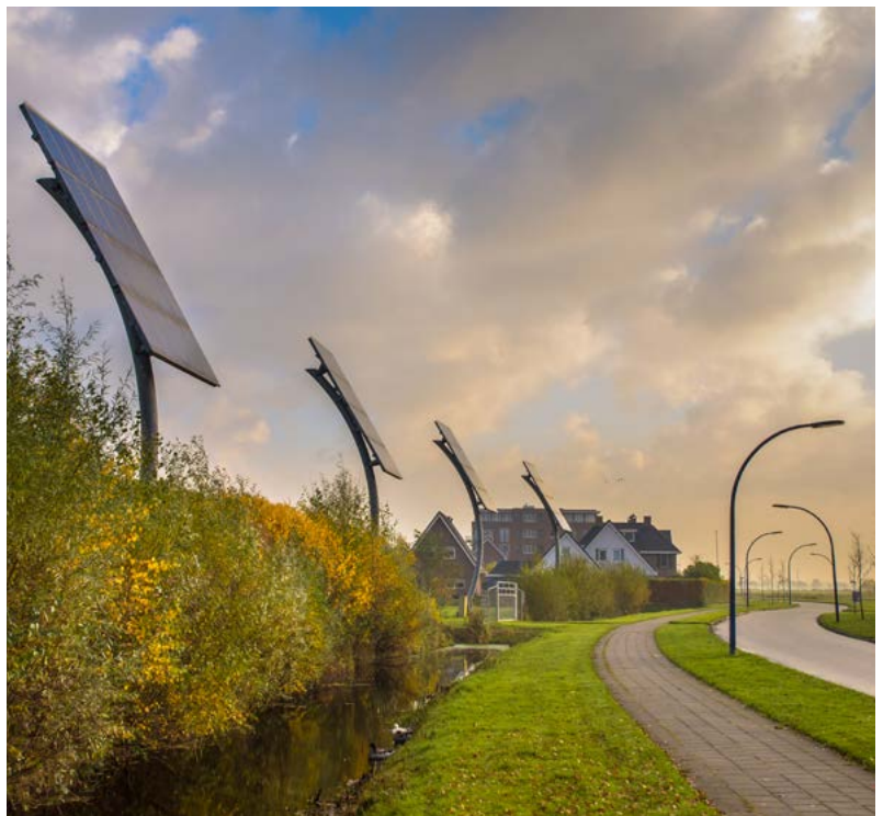
Local renewable energy scheme. Solar lighting along path in housing estate.
