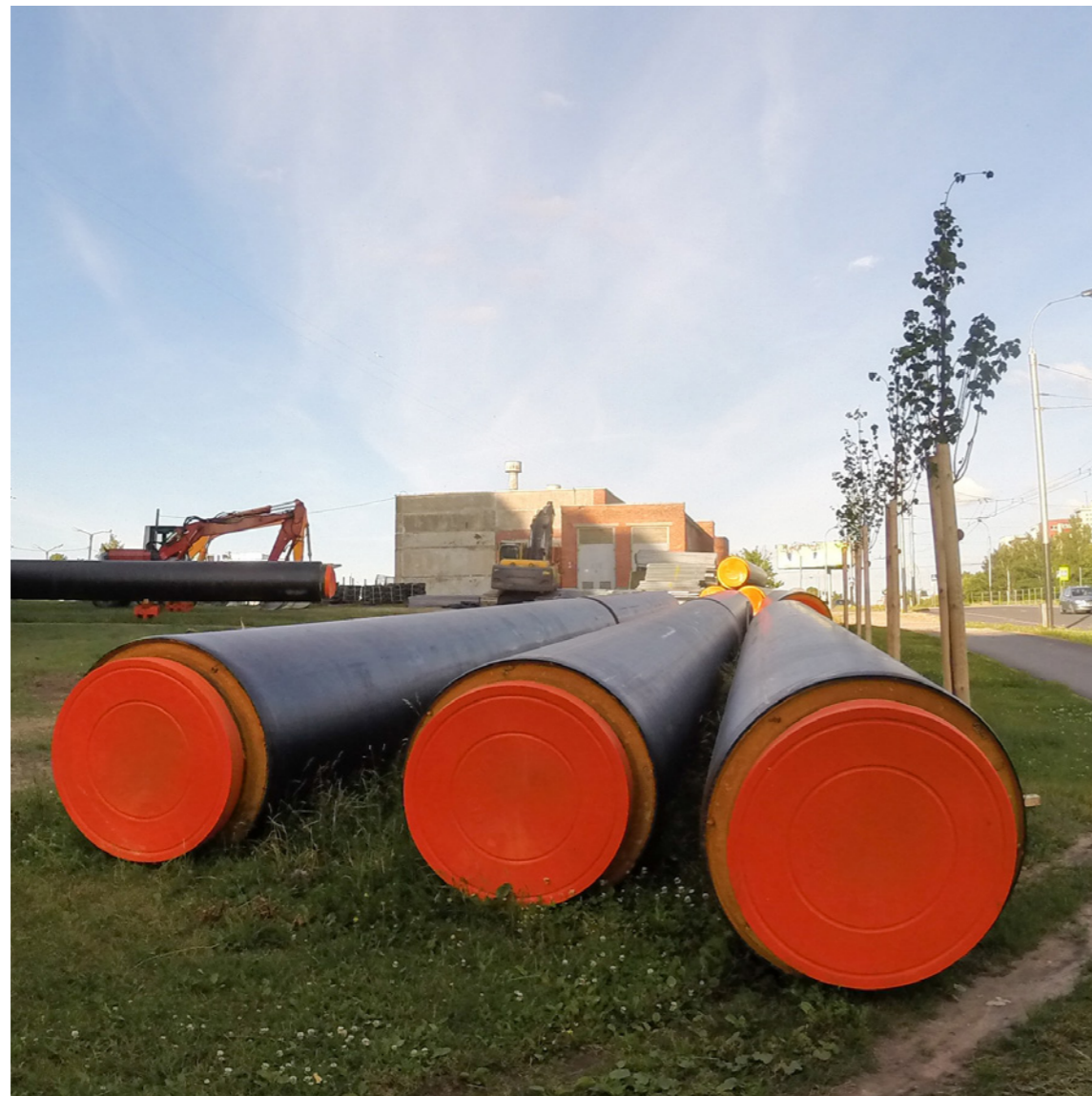
Pre-insulated district heating pipes ready to be laid
